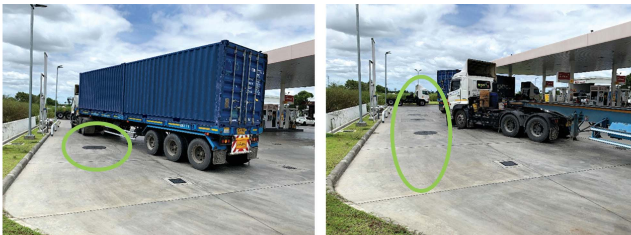
Figure 2 – Access covers in consideration of traffic flow
